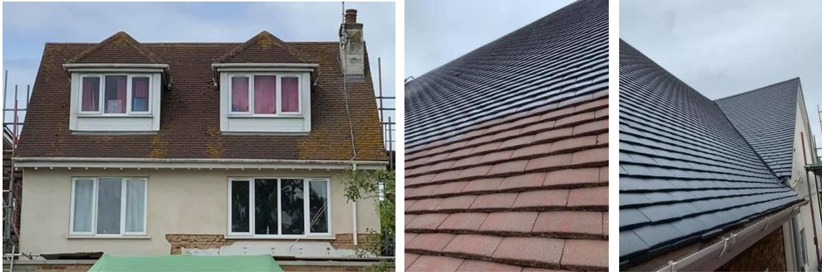
The process for the roof took nine days in total. It included a full clean, followed by a coat of Andura biocide, before finally applying two coats of Andura Roofgard in the colour 'slate grey'.
